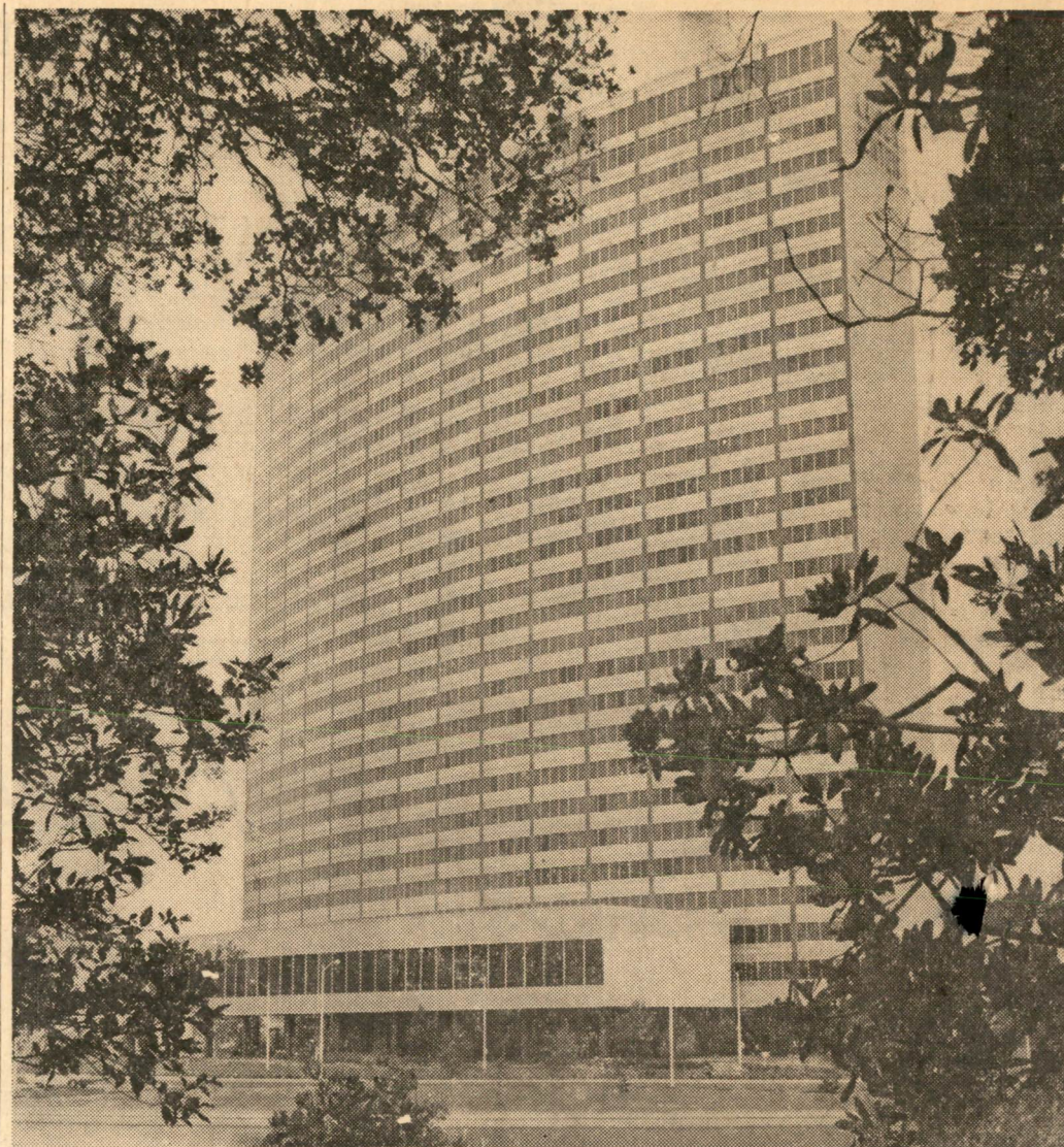
Built in the form of an arc to follow the gentle curve of the Lake Merritt shore line in Oakland, Calif., this 28 story building is the headquarters of 60 affiliated
