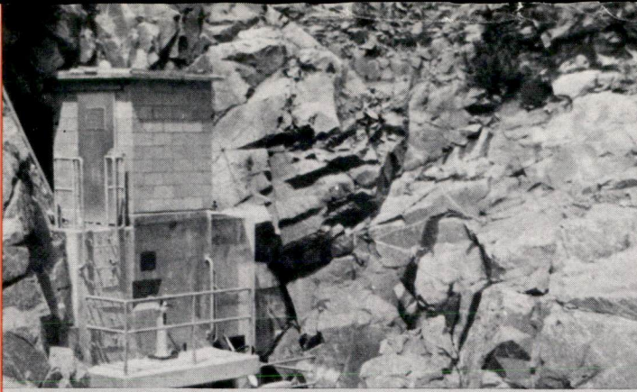
Lower Hell Hole Dam on the Rubicon River is owned by the Placer County Water Agency. A 400-kilowatt plant at this site could generate 3 million kilowatthours of electricity annually.
