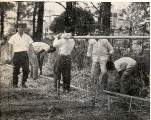
Villagers pitch in to lay pipe for a local water supply.
