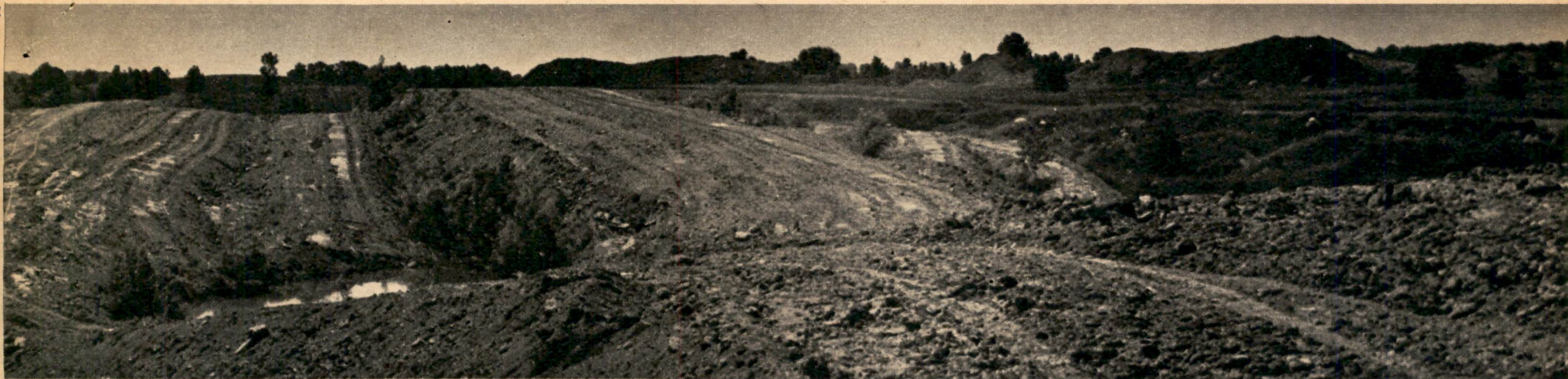
Bulldozer shapes spoil banks into rolling hills at United Electric Coal Co.'s Fidelity Mine near DuQuoin, Ill. The land is usually allowed to settle for a few years before grading and seeding process begins.
