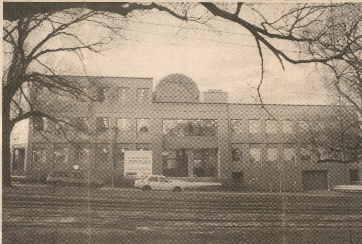
The building in Victoria Parade, Collingwood, leased by Telecom Mobile.
